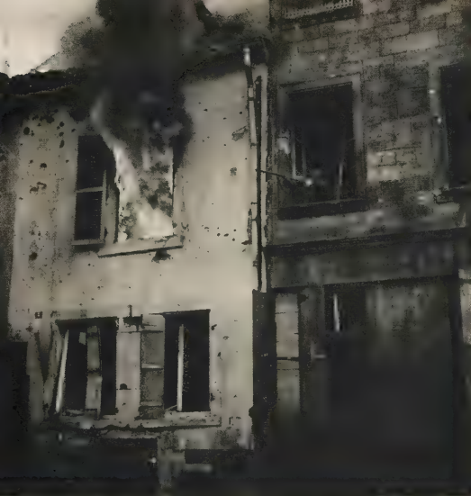
An 8th Div infantryman fires at Kraut snipers hiding on nearby rooftops in Brandenburg, while fire from exploding mortar shell burns in next building.
